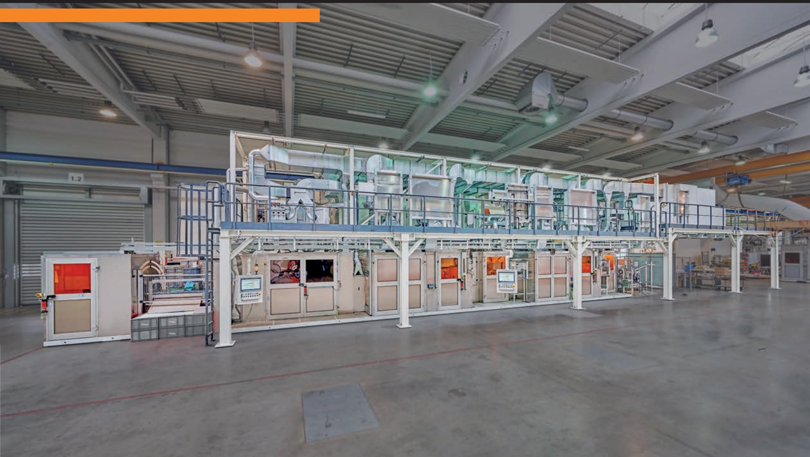
Plant for coating battery cells with UV-curable paint
